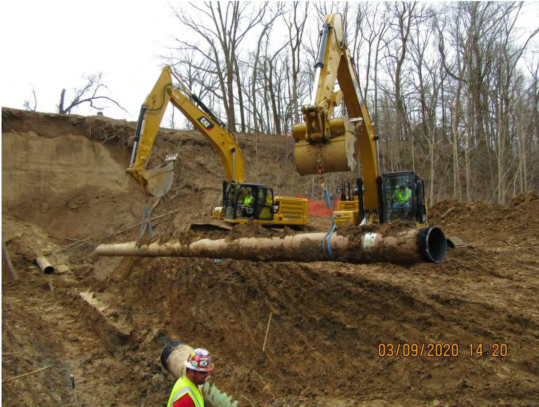
Figure 9. Upstream Pipe Section During Removal
