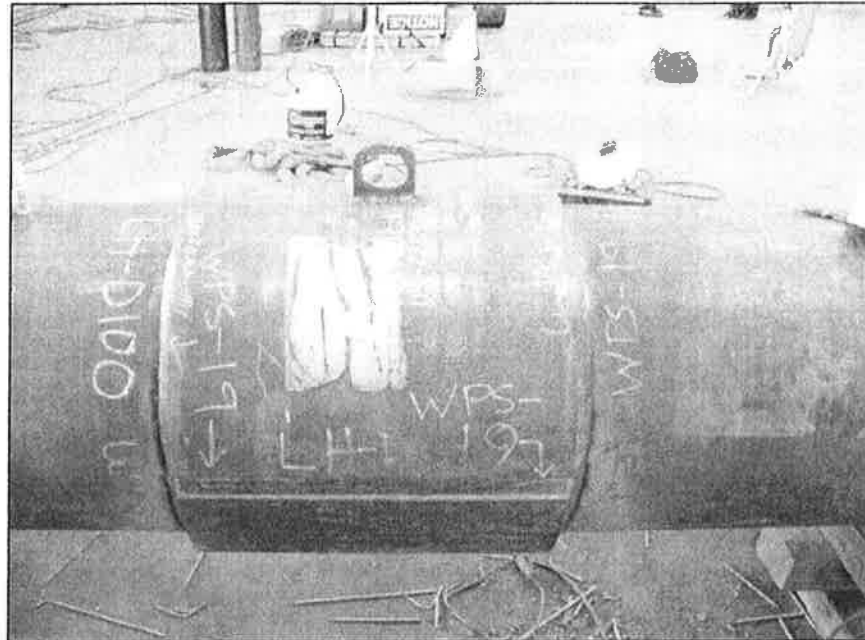
Figure 3. In-service tight-fitting repair sleeve.
